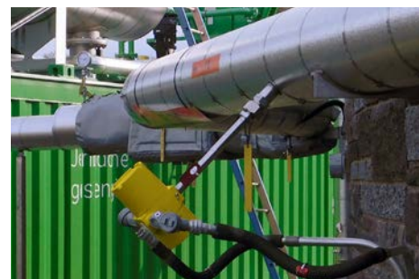
Figure 4. Consider meter flow straight-run requirements and flow disturbers.
