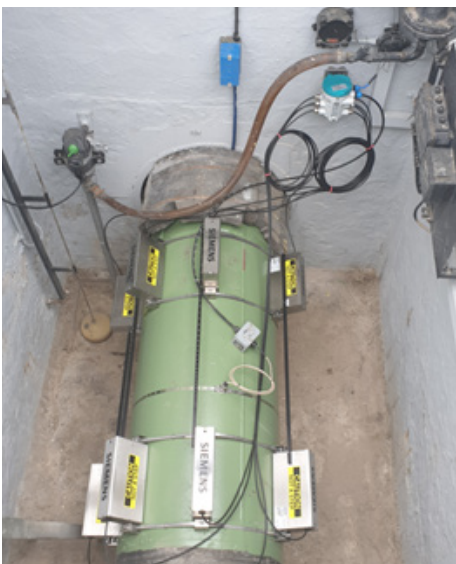
Figure 6: SITRANS FS230 measuring hydrocarbon liquids with 4 path installation of wide-beam SITRANS FSS200 sensors in reflect mode, clamp-on temperature sensor in Zone 0, external DSL in Zone1 and wall mounted SITRANS FS230 about 100 meters away in Zone 2 hazardous area.
