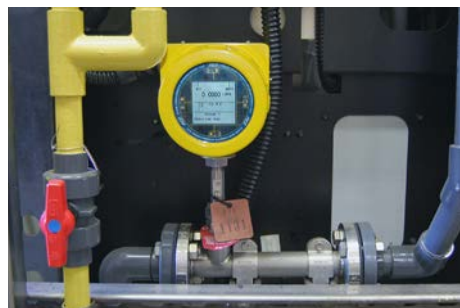
Figure 4. Consider meter flow straight-run requirements and flow disturbers.
